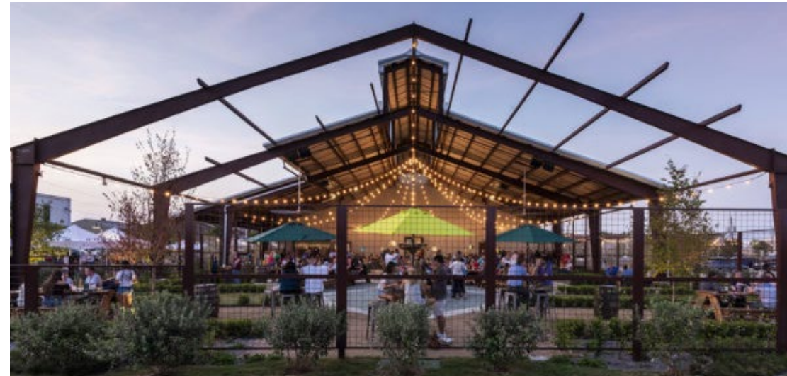
Restaurant Building with Outdoor Patio
